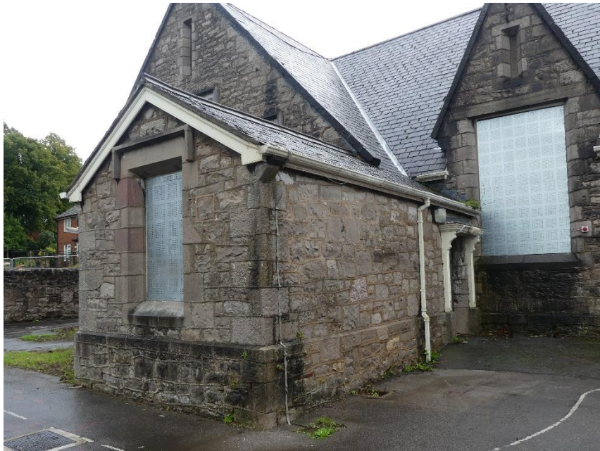
Figure 4.22: Detail of the front porch
