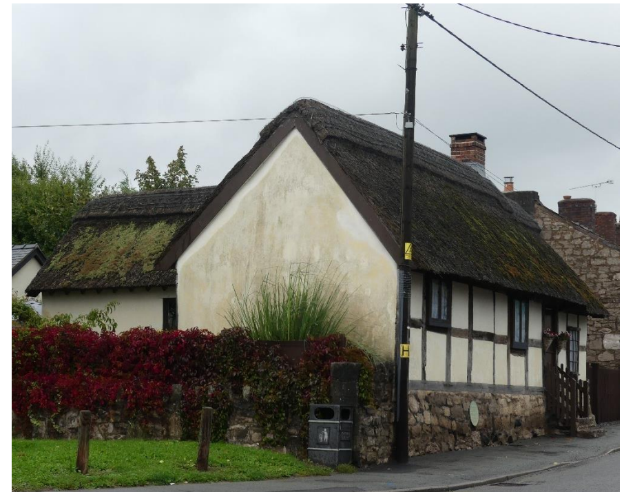
Figure 4.3: The front elevation and west gable of Rose Cottage
