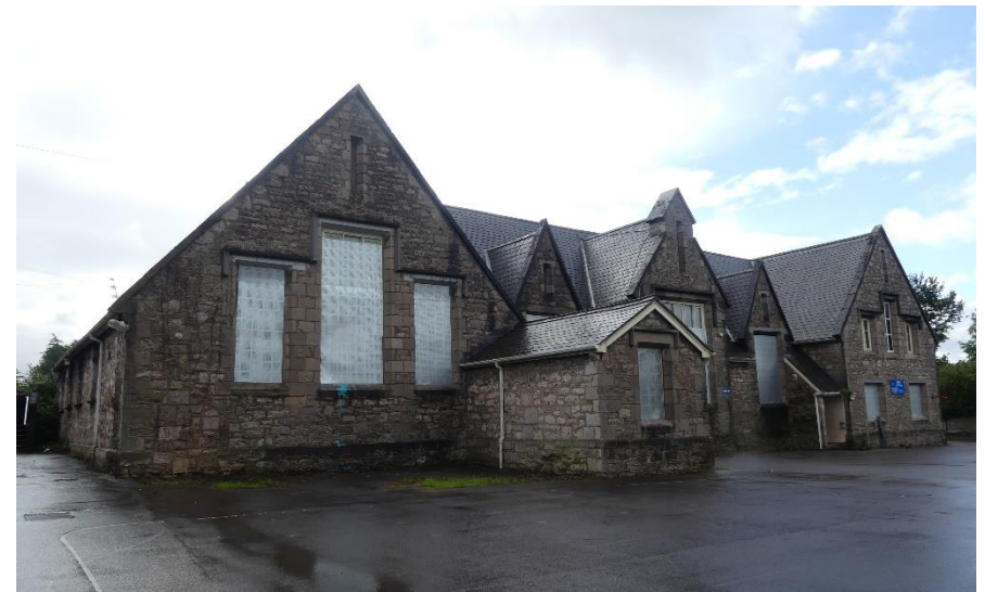
Figure 4.21: The front elevation of Ruthin British School
