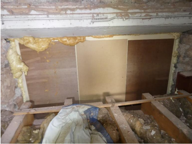
Figure 4.30: A window head concealed within the roofspace
