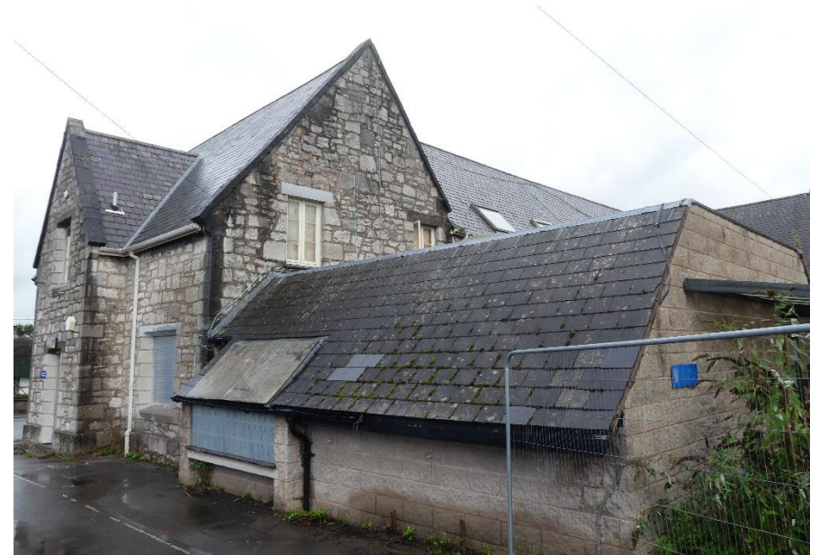
Figure 4.23: The western elevation and associated extension
