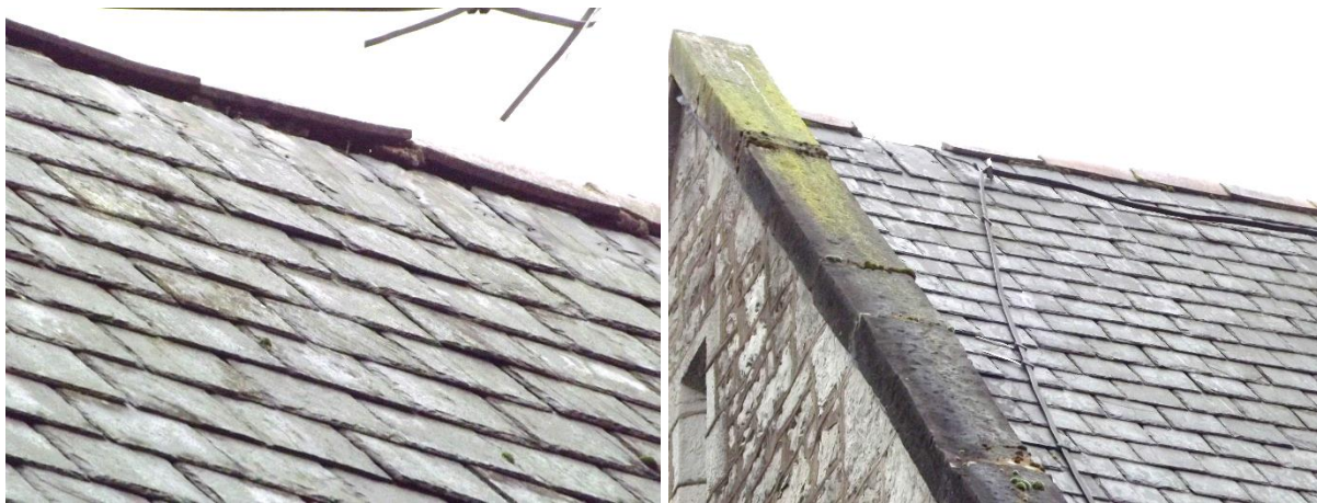
Figure 6. Lifted ridge tiles (left), missing ridge tiles and loose slates (right)
