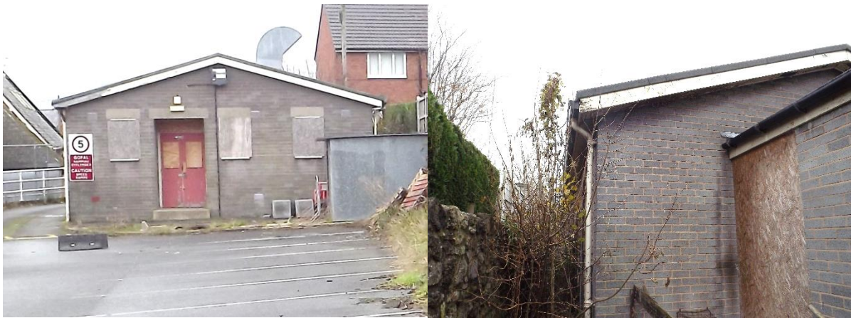
Figure 9. South elevation and entrance (left), north elevation and flat roof extension (right)
