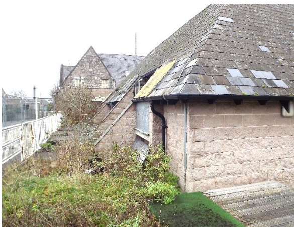
Rough grassland bordering west side of building B
