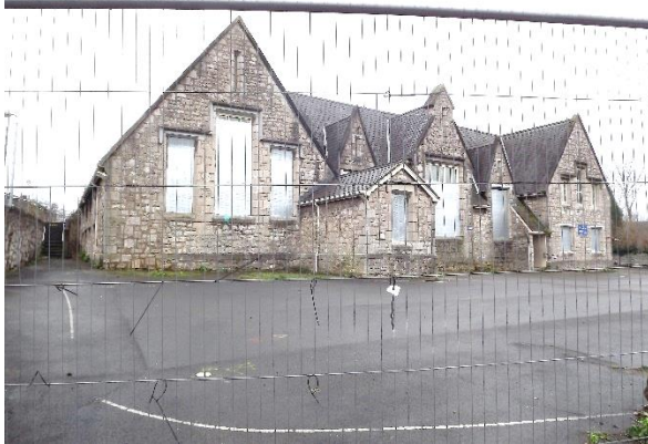
Building A and tarmac playground
