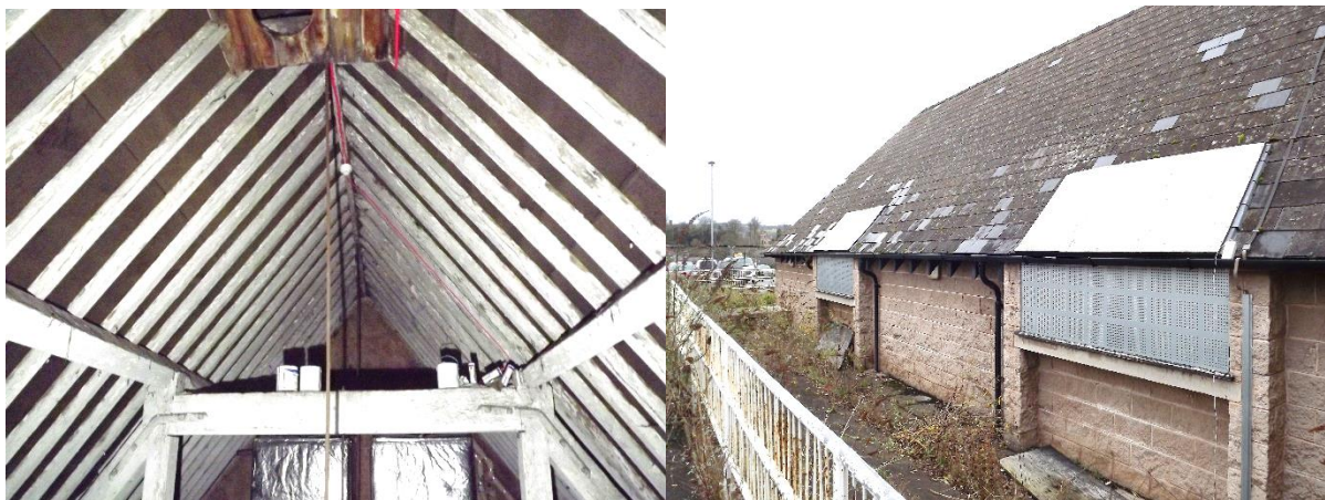
Figure 7. Roof space (left), south elevation (right)
