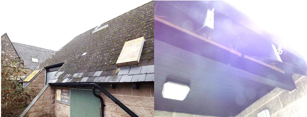
Figure 8. West roof elevation (left), voids beneath the overhanging roof (right)
