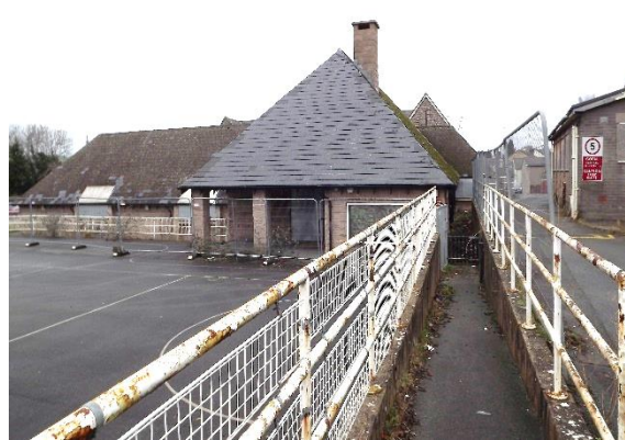
Building B and tarmac playground and path
