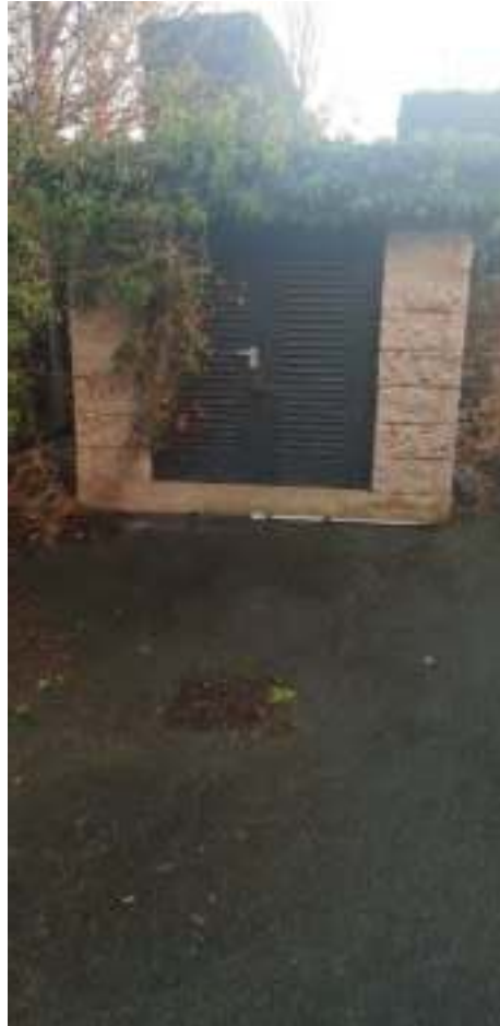
Electricity Substation in the east of the site.
