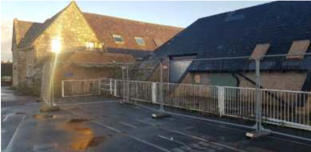
Original school building in the background with modern extension in the foreground. Photo looking northeast from western boundary.
