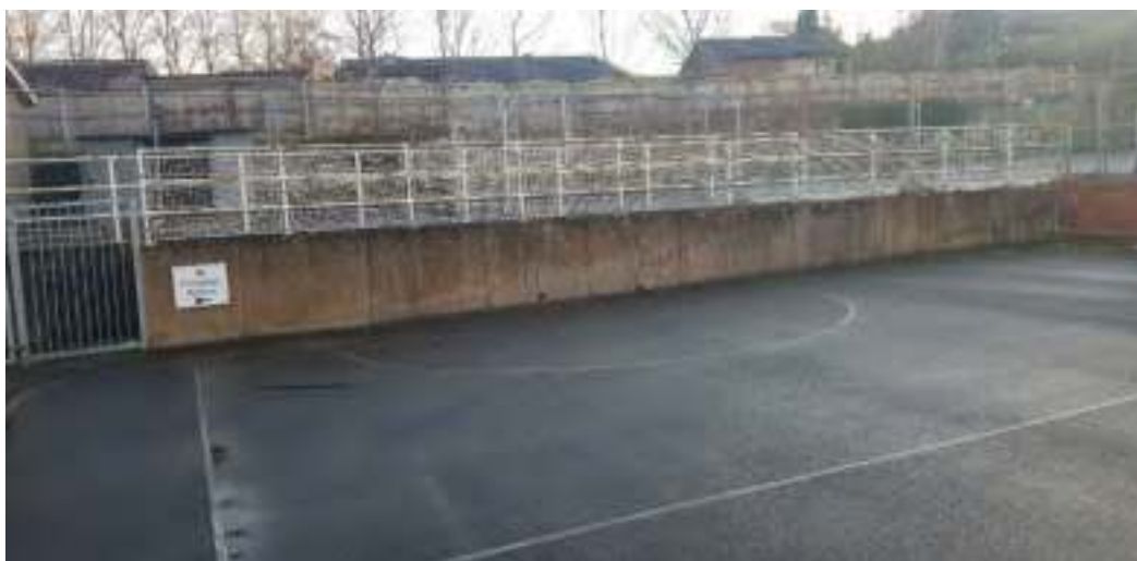
Concrete retaining wall in the east of the site supporting access road to car park located to the south of the playground.
