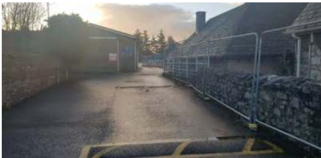
Current vehicular access off Rhos Street along eastern boundary of the site, with main school building approximately 1m below road level.
