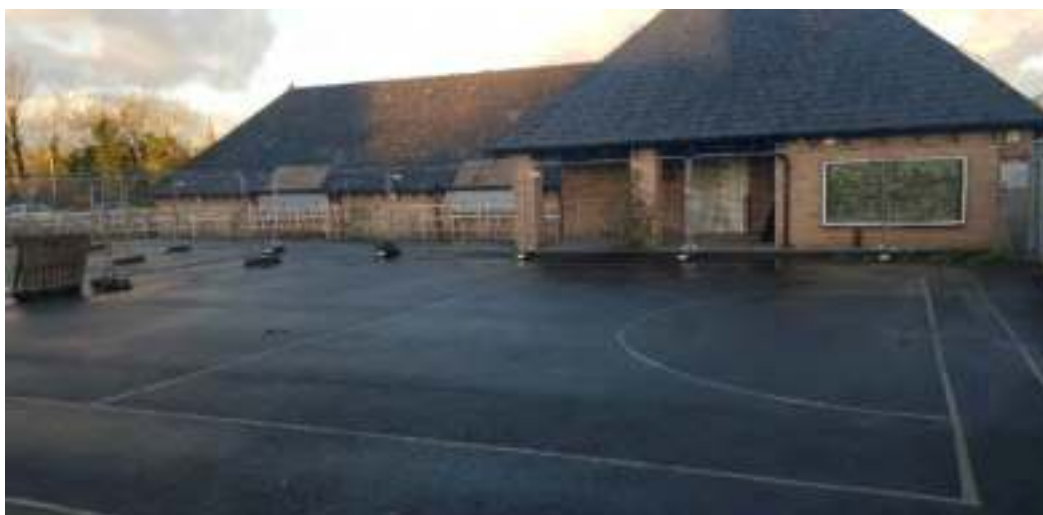
View from the south across playground to modern extension
