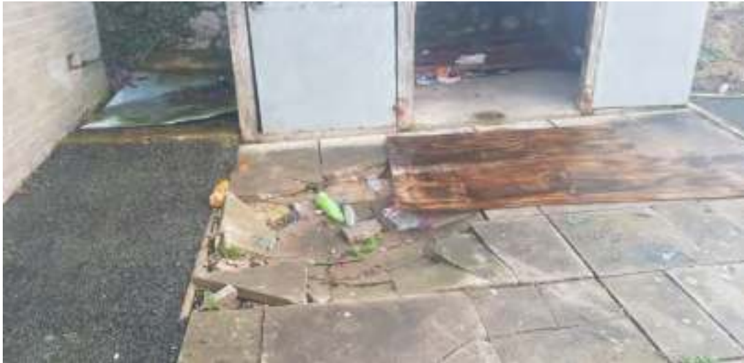
Collapsed paving in the east of the site to the north of the community building.
