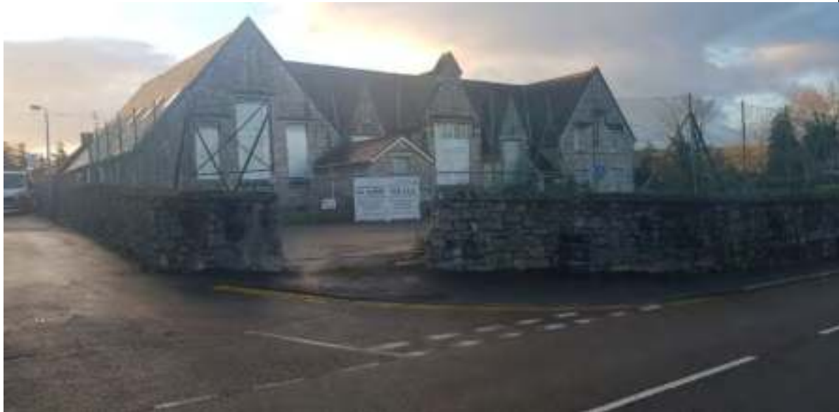
Existing site entrance from Rhos Street, with original school building in the background.
