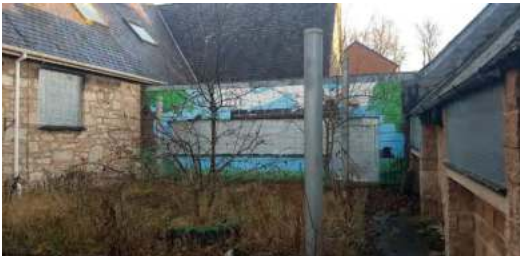
Courtyard area between the original school building to the left and newer extension to the right. Steel posts supporting former sun canopy.
