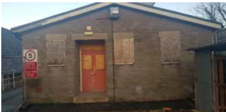
Former community building in the east of the site.
