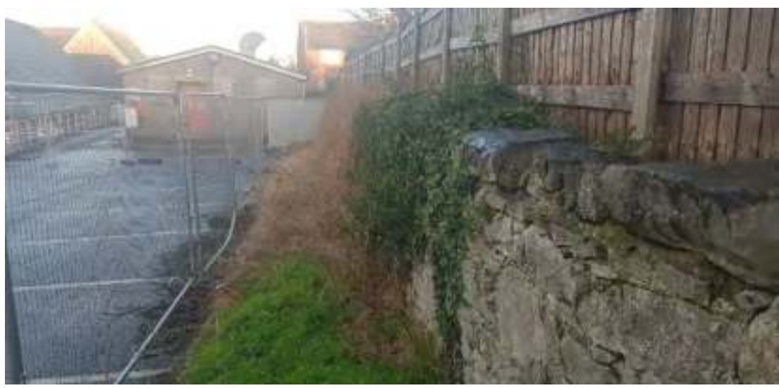
Stone retaining wall along eastern boundary, looking north.
