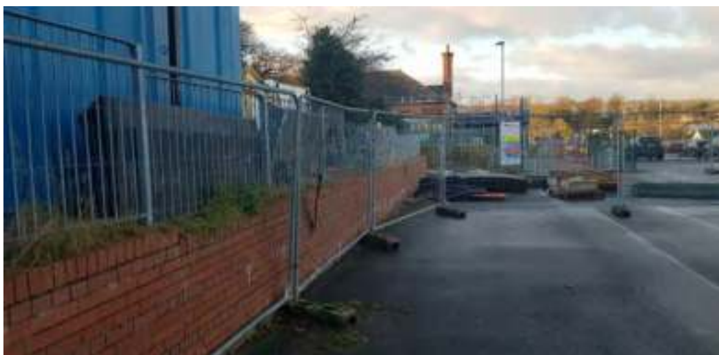
Brick retaining wall supporting car park above playground.
