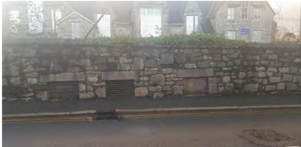
Existing Rhos Street retaining wall with three openings, with original school building in the background.
