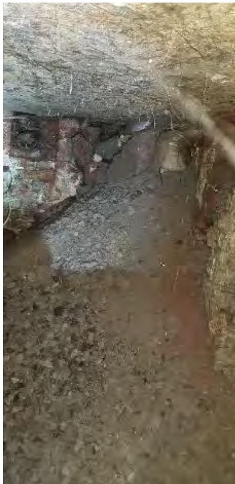
Possible former steps into basement feature, filled with lean mix/aggregate.
