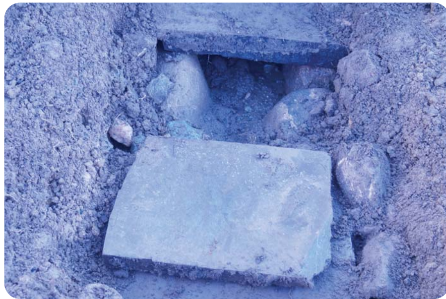
Plate 6. Trench 2 - Land Drain Slate Capping Slabs and Stone Sides
