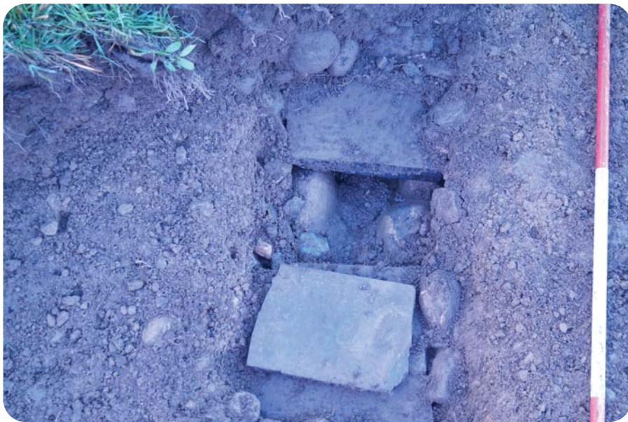
Plate 5. Trench 2 - Land Drain Slate Capping Slabs and Stone Sides
