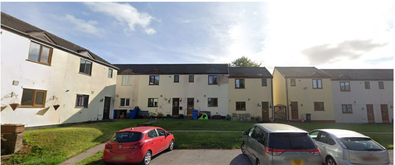
Photos of existing adjacent residential cul-de-sac
